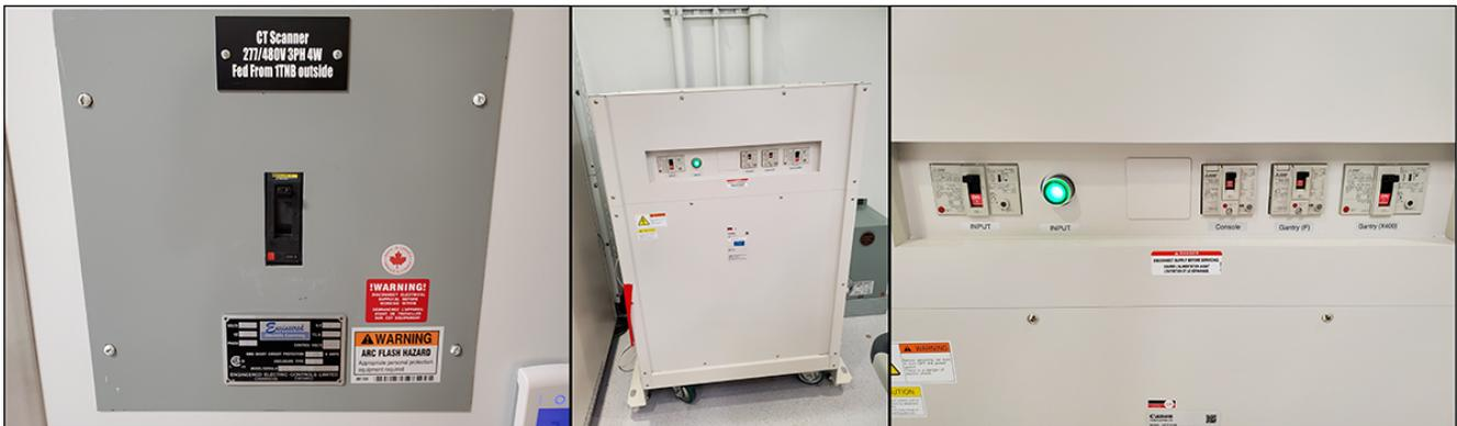
6. Occasionally, the gantry switch may be tripped after outage. It is located on the backside of the scanner on the lower left corner.
